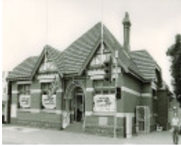
B5072 Former Shire Hall
