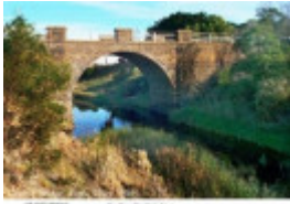
B2782 Grant's Bridge
