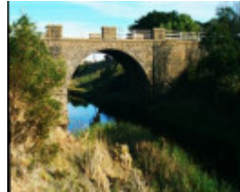
B2782 Grant's Bridge
