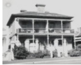
B3414 19-21 Alfred Crescent Fitzroy North
