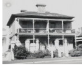
B3414 19-21 Alfred Crescent Fitzroy North
