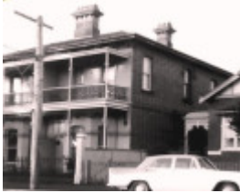
B3414 19-21 Alfred Crescent Fitzroy North
