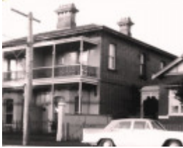
B3414 19-21 Alfred Crescent Fitzroy North
