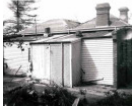
B3520 Cleveland Rear View
