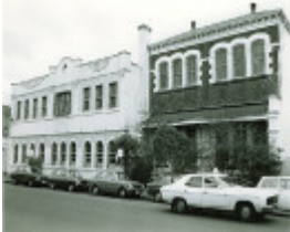
B4506 Bell St Special School 38 Bell St Fitzroy
