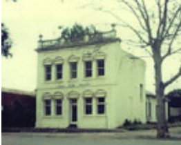
B5473 Former Colonial Bank
