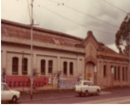
B4138 Fmr Cable Tram Depot
