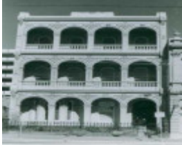
B3297 The Terrace 11 Brunswick St Fitzroy
