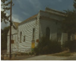
B5448 Former Mechanics Institute
