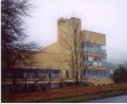
b4918 Sanitarium Factory Complex Main St Warburton
