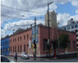
B6431 Fmr Fitzroy Cable Tram Engine House
