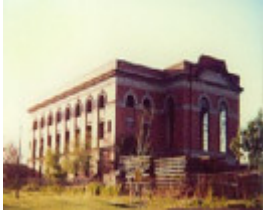
B5903 Former Substation
