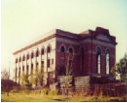
B5903 Former Substation
