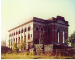
B5903 Former Substation
