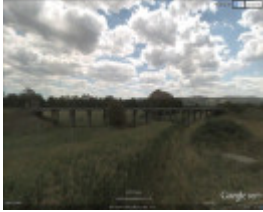
B7069 Stringybark Creek Bridge
