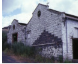
1 former melbourne meat preserving company building van ness ave maidstone end view dec1981
