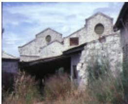
former melbourne meat preserving company buildings van ness ave maidstone side elevation dec1981
