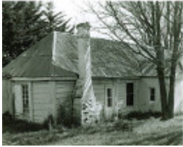
B2400 Slab Cottage Yarra Glen
