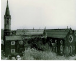
B3718 St Joseph's Building
