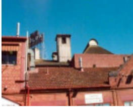
B7204 Cremorne Malting Building
