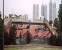
B7125 Nth Fitzroy Railway Footbridge
