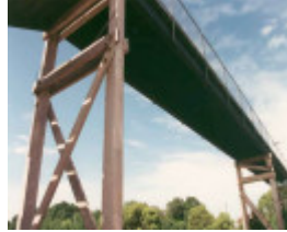
B7125 Nth Fitzroy Railway Footbridge
