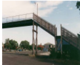
B7125 Nth Fitzroy Railway Footbridge
