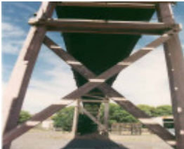
B7125 Nth Fitzroy Railway Footbridge
