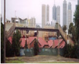
B7125 Nth Fitzroy Railway Footbridge
