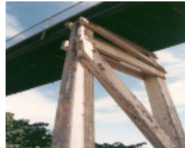
B7125 Nth Fitzroy Railway Footbridge
