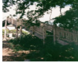
B7125 Nth Fitzroy Railway Footbridge
