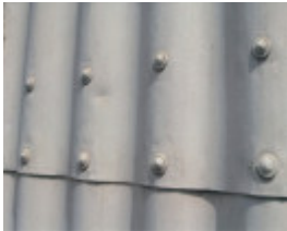
67162 B5311 Iron Store detail NW facade
