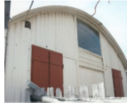
67162 B5311 Iron Store SW facade
