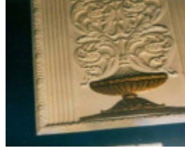
B6994 Fmr Clifton Cinema Wall Detail
