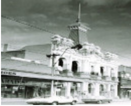
B5010 Former Post Office
