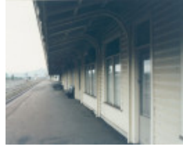
B6679 Railway Station Complex
