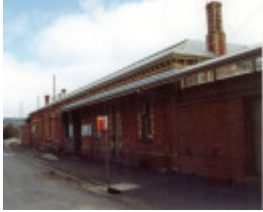
B6679 Railway Station Complex
