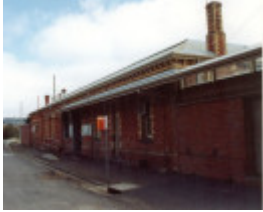
B6679 Railway Station Complex
