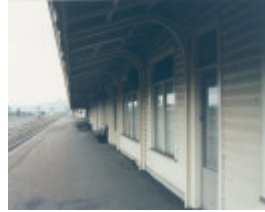
B6679 Railway Station Complex
