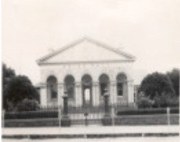
B2117 Former Shire Hall
