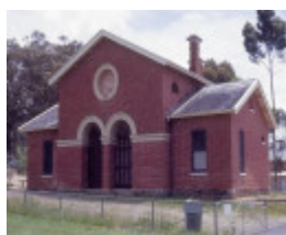
h01652 former maldon court house fountain street maldon front south east she project 2003
