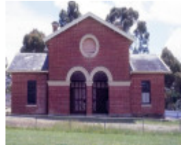
h01652 1 former maldon court house fountain street maldon front she project 2003
