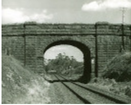
B3166 Navigators Railway Bridge
