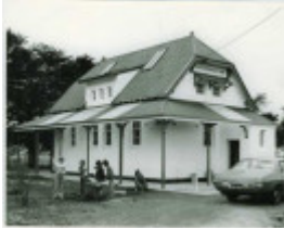
B3871 Former Cardigan Primary School
