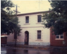
B5590 Former Manager's Residence
