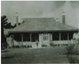
B2153 Mine Manager's Residence
