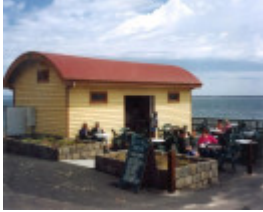
B6464 Jetty Shed
