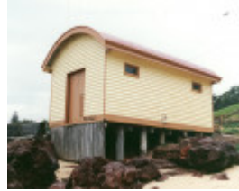
B6464 Jetty Shed
