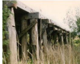
B6945 Lang Lang River Bridge
