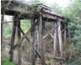
B6945 Lang Lang River Bridge
