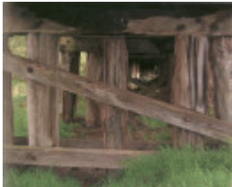
B6945 Lang Lang River Trestle Bridge
