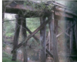
B6945 Lang Lang River Trestle Bridge
