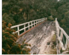
B6923 Springdallah Bridge
