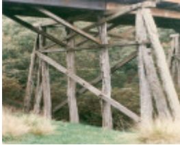
B6923 Springdallah Bridge
