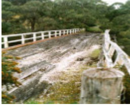
B6923 Springdallah Bridge
