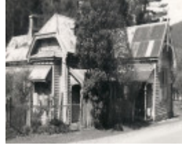
B3248 Post Office & Residence
