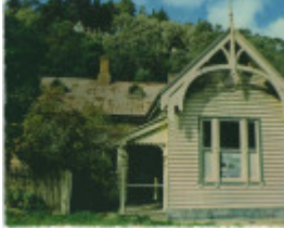
B3248 Post Office & Residence
