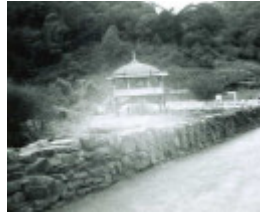
B3552 Stone Retaining Walls
