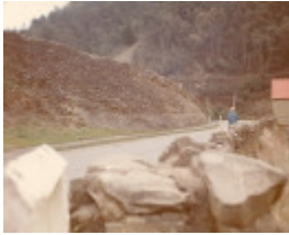
B3552 Stone Retaining Walls
