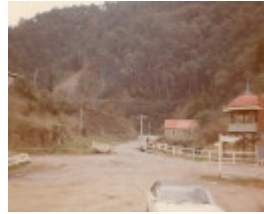
B3552 Stone Retaining Walls
