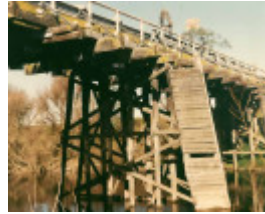
B0287 Calulu Bridge
