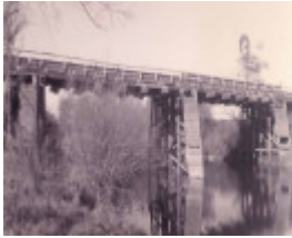
B0287 Calulu Bridge
