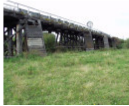
B0287 Calulu Bridge
