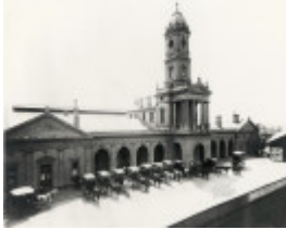
B0276 Ballarat Railway Station
