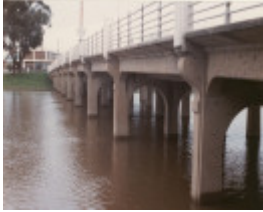
B5744 Concrete Girder Road Bridge
