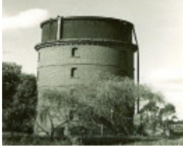
B2650 Water Tower
