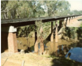
B5746 Rail Bridge
