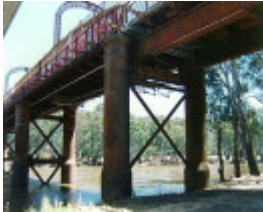
B2091 Echuca Bridge over Murray River
