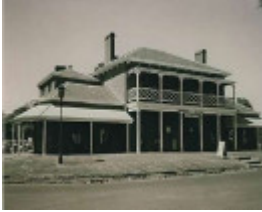
B1327 Bridge Hotel
