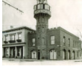
B3282 Former Ballarat Fire Station
