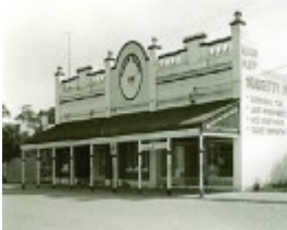
B4766 Glasgow Buildings
