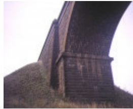
rail bridge over coliban river malmsbury detail of arch apr1995
