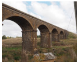
MALMSBURY RAIL BRIDGE 2020
