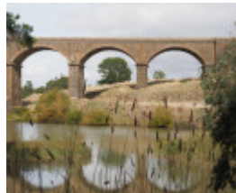
MALMSBURY RAIL BRIDGE 2020
