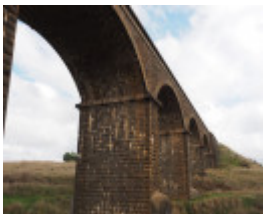
MALMSBURY RAIL BRIDGE 2020
