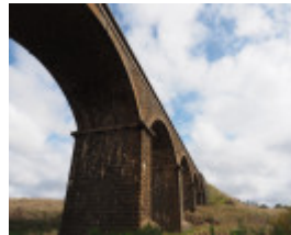
MALMSBURY RAIL BRIDGE 2020
