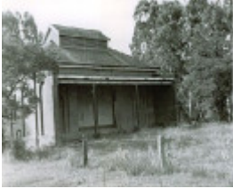
B1311 Pumping station
