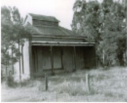
B1311 Pumping station
