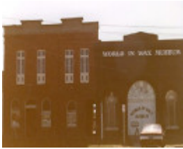
B4178 Former Shackell's Bond Store
