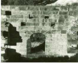
B2080 Entrance Arch Duke & Timor Mine
