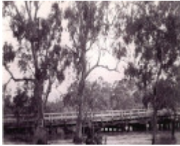
B6843 Archdale piers
