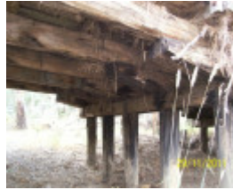
B6843 Archdale substructure
