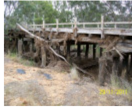
B6843 Archdale Bridge
