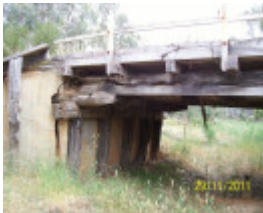
B6843 Archdale abutment
