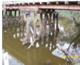
B6843 Archdale Bridge
