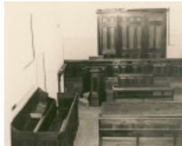
B2750 Courth House Interior1
