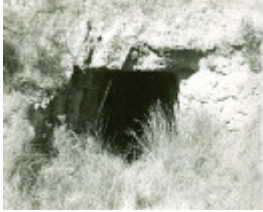
B2712 Mine Tunnel
