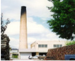
B6451 Boiler House Maryborough & District Hospital
